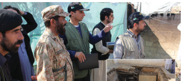
KP Malakand Division 31 Oct, 2015: NDMA Teams conducting damage assessment for compensation verification process at village Killa Pata, U.C Malanjaba, Tehsil Charbagh, District Swat.
